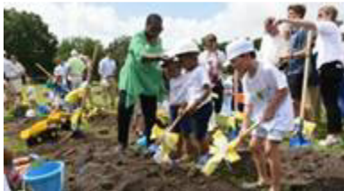
May 2017 Groundbreaking for the new Louisiana Children's Museum in New Orleans City Park.
